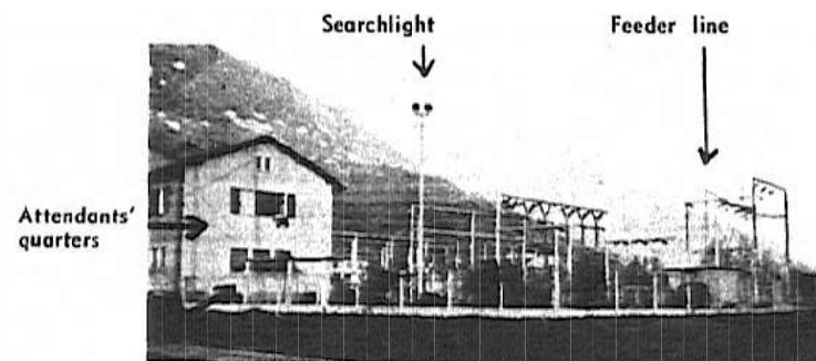
Overall view of a transformer station
