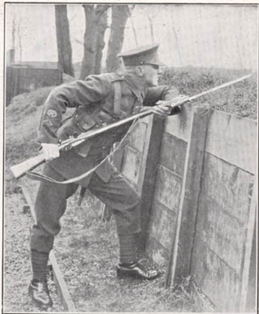
USE OF COVER. TRENCH. POSITION OF READINESS.
