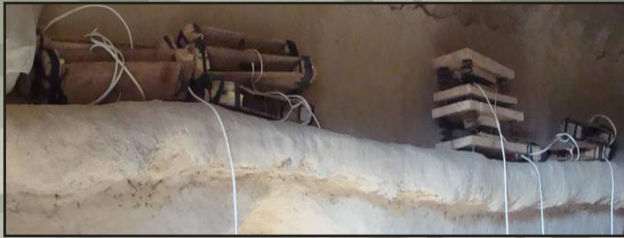
Cache -Various PPs Under Construction
