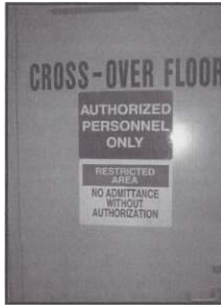
Crossover floors, whatever their signs may warn, should be unlocked in compliance with fire codes. They're good routes out of stairwells.
