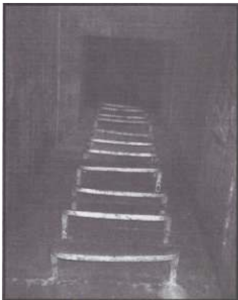
Stepirons set into the concrete at the side of the drain are often used in place of ladders.
