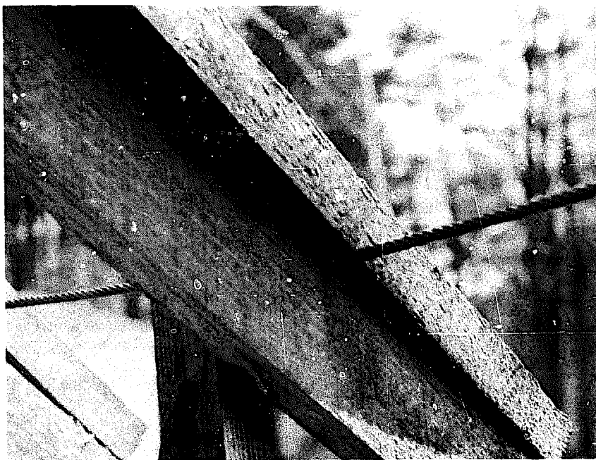
Sandwiching the cable between roof pieces; nail above the cable itself.
