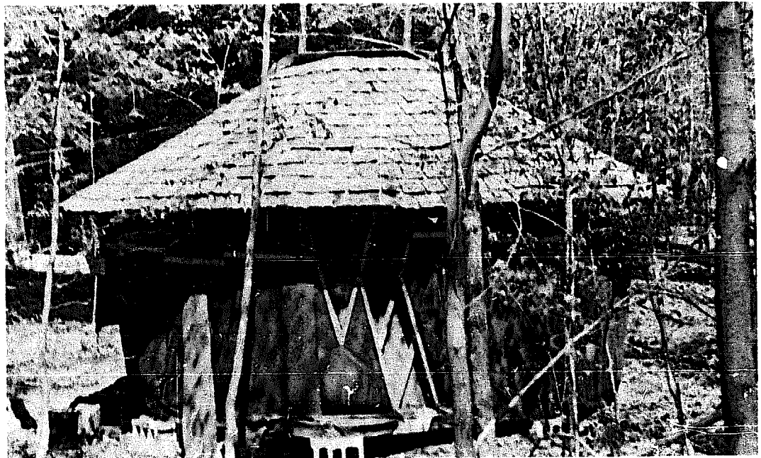
CUTTING DOORS AND WINDOWS
