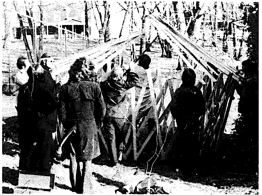
Pole method of supporting roof pieces.
