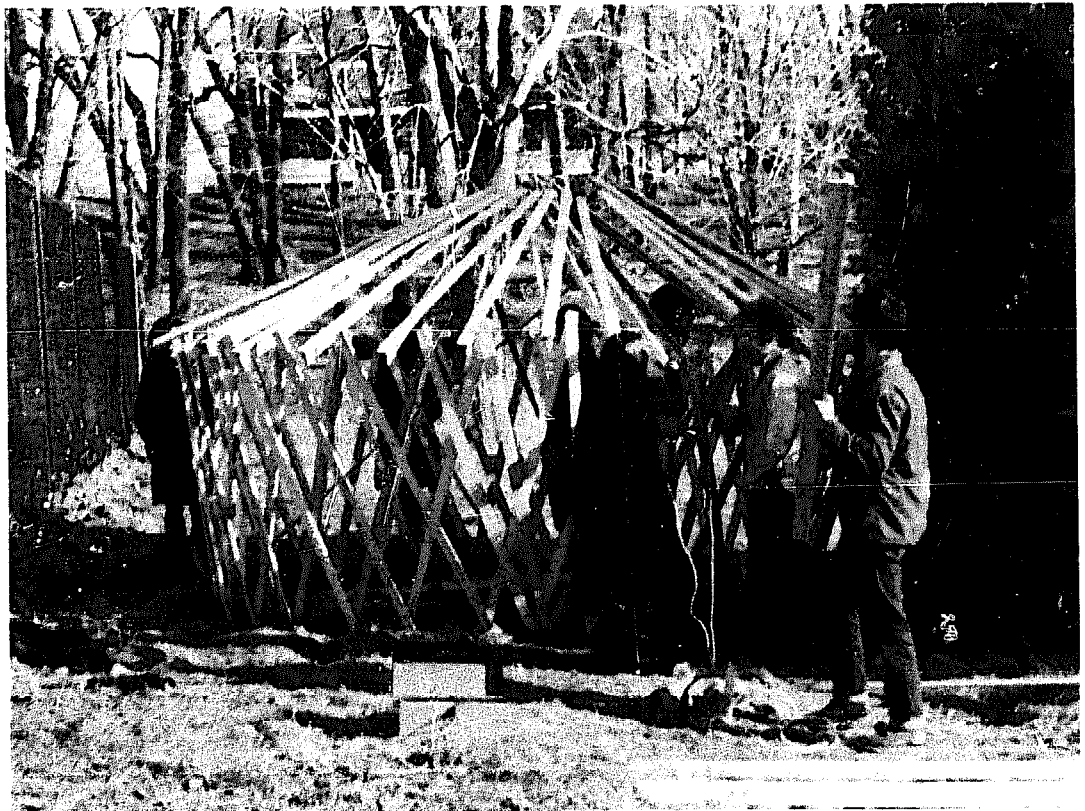
Roof assembly in progress.
