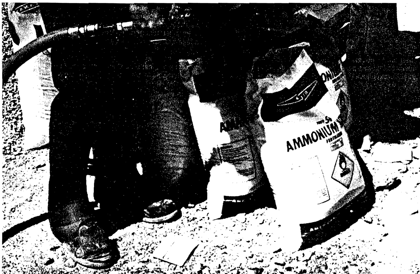
Figure 16.—Field mixing of AN-FO. (Courtesy Hercules Inc.)
