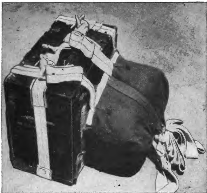
FIGURE 8. —Type A-7 ammunition delivery unit with canopy in pack preparatory to dropping.
