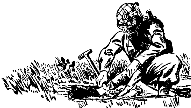
SPOIL BEING REMOVED CORRECTLY
