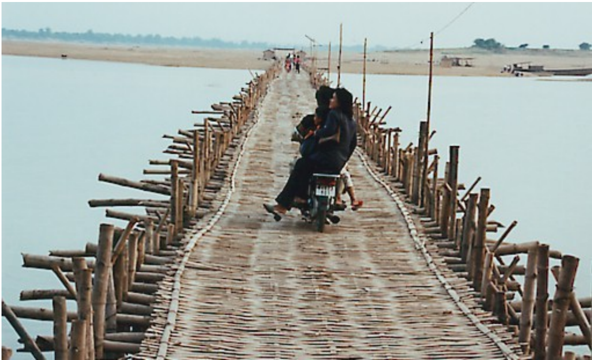
This bamboo bridge runs from the mainland to an Island, where the locals grow produce. Believe it or not, the bridge, which can support heavy cars and trucks, is dismantled every rainy season, to keep it from being washed away.
