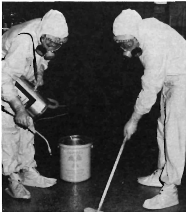
A professional decontamination team at work. Although workers are taking elaborate pains to see that no radioactive material touches them, the fundamental activity is no more complex than scrubbing the floor. (Photograph courtesy of Nuclear Associates, Inc., 100 Voice Road, Carle Place, New York 11514.)
