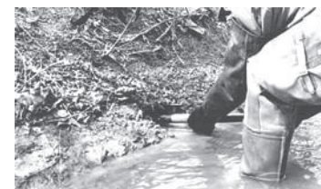
Dig pocket at water line.
