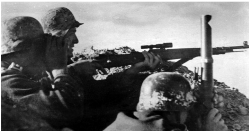
A German sniper. The small size and long eye relief of the 1.5× Zf 41 telescopic sight is very apparent in this view. It essentially attached to the rear-sight base, rather than mounting over the receiver as in the case of the larger-magnification sights. This photo is almost certainly a posed shot; although the man to the shooter's right is using an observation periscope, his two comrades exposing their heads rather defeats the point. (Tom Laemlein/Armor Plate Press)
