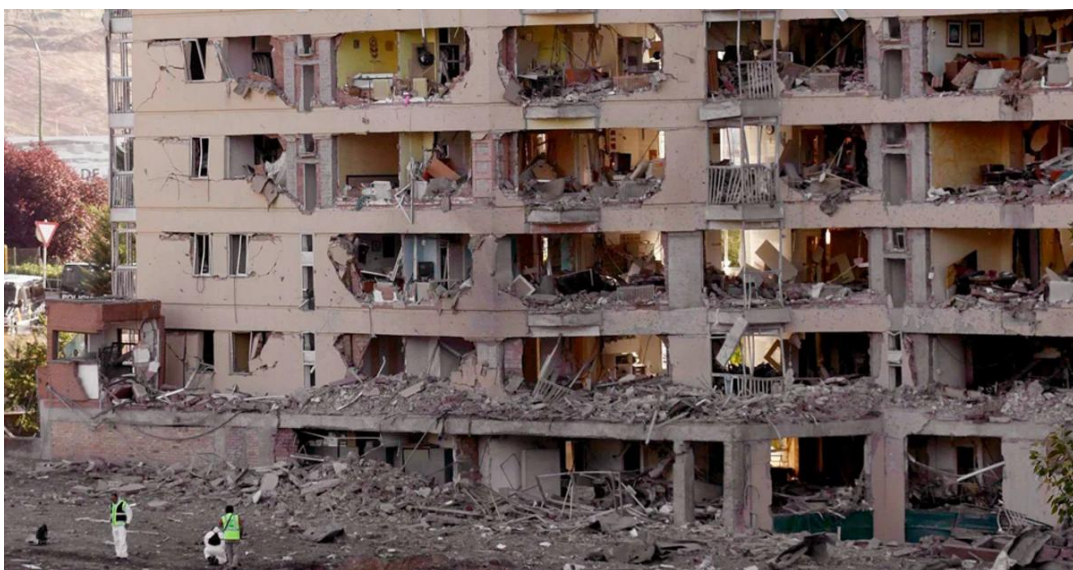
1987. Zaragosa, Spain. 11 dead, 88 injured. 250 kg ammonal.
