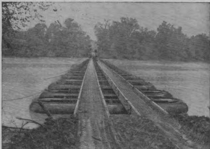
FIGURE 121.—Steel treadway bridge.
