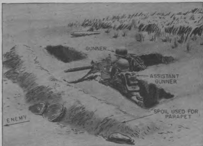
FIGURE 65.—Caliber .30 machine-gun (light) emplacement, fox-hole type.
