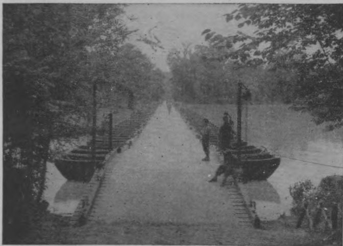
FIGURE 120.—Ponton bridge, 25-ton.
