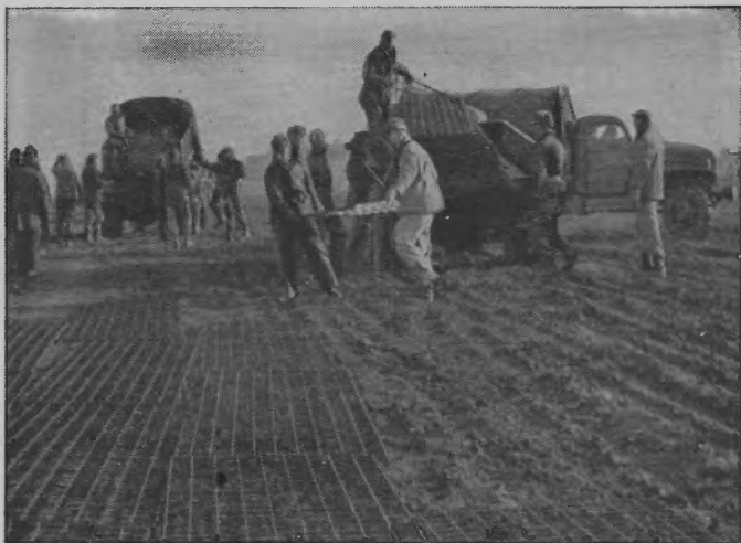
FIGURE 139.—Laying bar-and-rod type steel runway.
