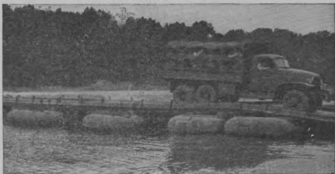
FIGURE 122.—Pneumatic bridge.
