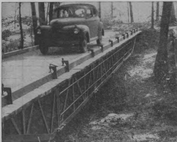
FIGURE 117.—Light portable steel bridge (H-10).
