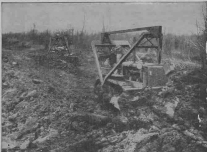
FIGURE 143.—Clearing and grading runway using bulldozers, typical pieces of heavy aviation engineer equipment.
