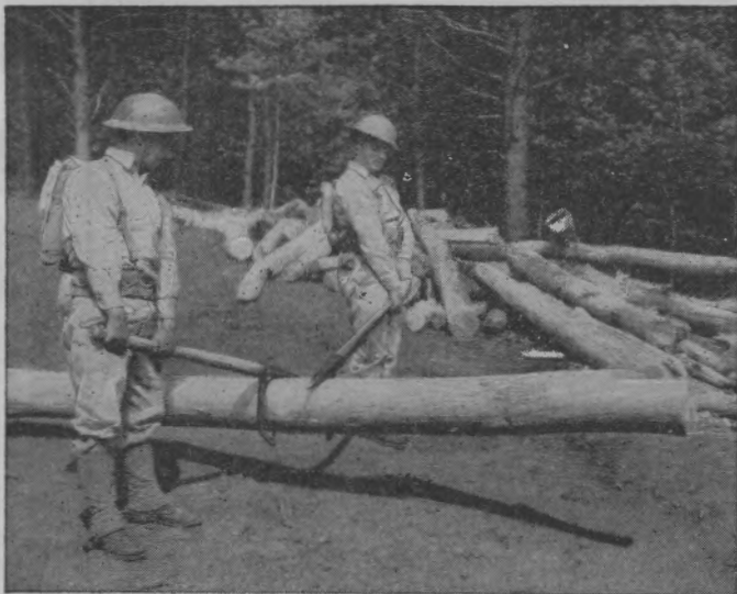
FIGURE 40.—Using the peavy to carry heavy timber.
