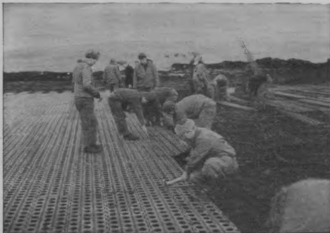
FIGURE 137.—Laying pierced plank steel runway.
