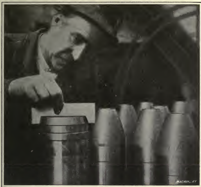
Fig. 91. Gaging Angle on Base End of Shell
