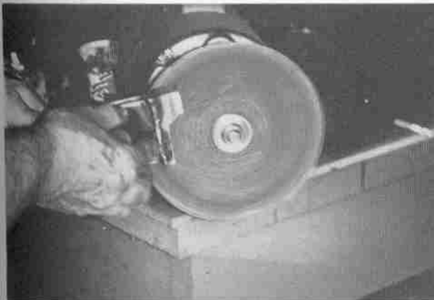
Welds are ground flush with disk sander.
