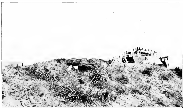
This illustration shows many points to be avoided. Nearly everything is wrong. The trench is located against the skyline, and no background has been placed behind the trench to prevent the heads of the occupants from being silhouetted against the sky. No attempt has been made to close the loophole with sandbags when not in use. The partly demolished building in the rear would furnish an excellent marker for the enemy's artillery.
