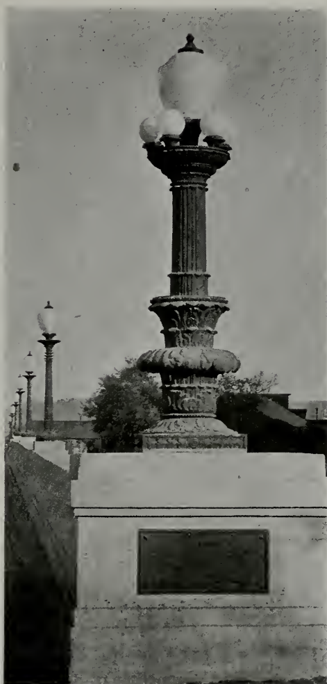
ELECTROLIER, WATSONVILLE BRIDGE
